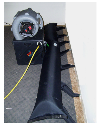
End opened for increased airflow
